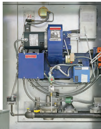
Figure 3 - Gas Burner
