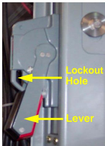
Figure 1-4 Flanged Disconnect Switch (side view)
