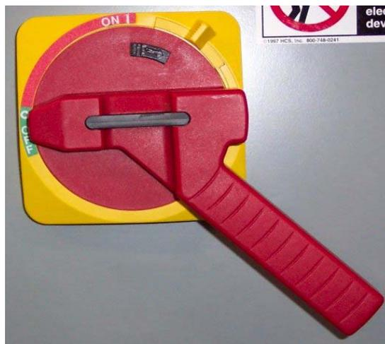
**Figure 1-2 Rotary Disconnect Switch (with longer handle)**
