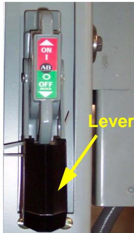
Figure 1-3 Flanged Disconnect Switch (front view)
