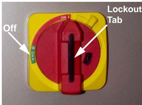
**Figure 1-1 Rotary Disconnect Switch**
