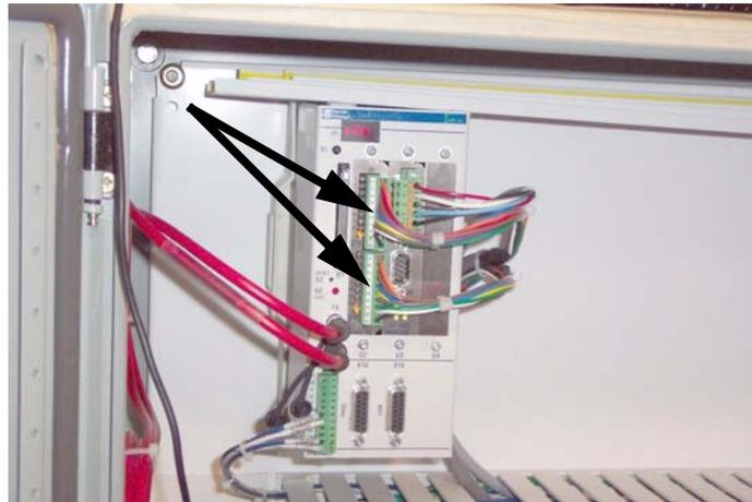
**Figure 2-4: Programmable Limit Switch in Servo Controller**
