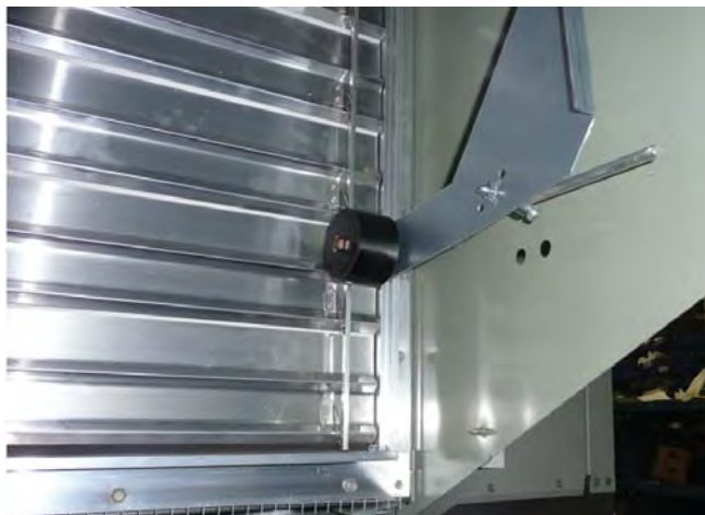
Figure 52. Exhaust damper linkage arm
