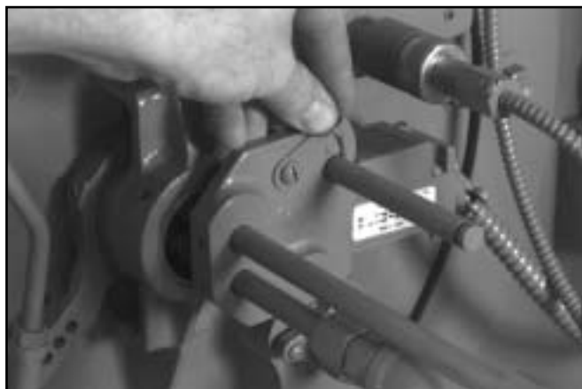
Figure: 5-9 Gun Locked In, Firing Oil
