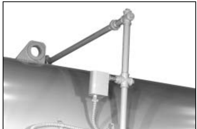
Figure: 1-13 Low Water Cutoff (LWCO Hot Water)
