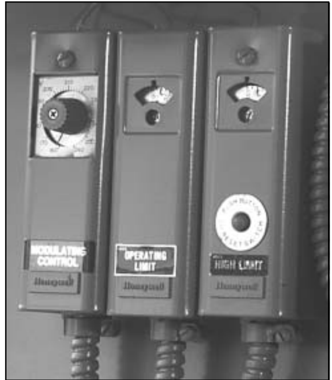
Figure: 1-12 Hot Water Controls
