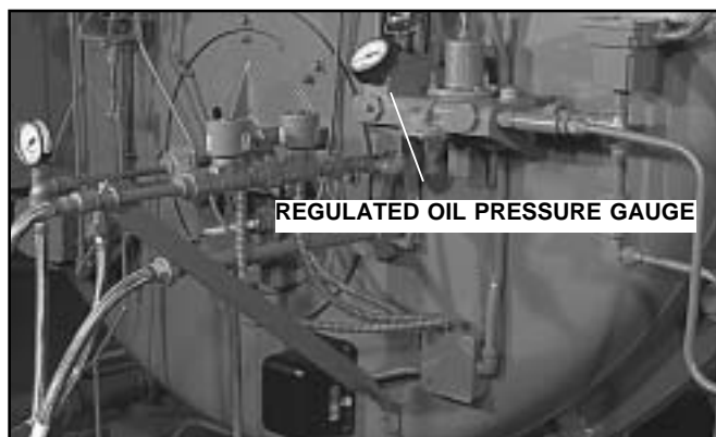
Figure: 5-8 Oil Piping
