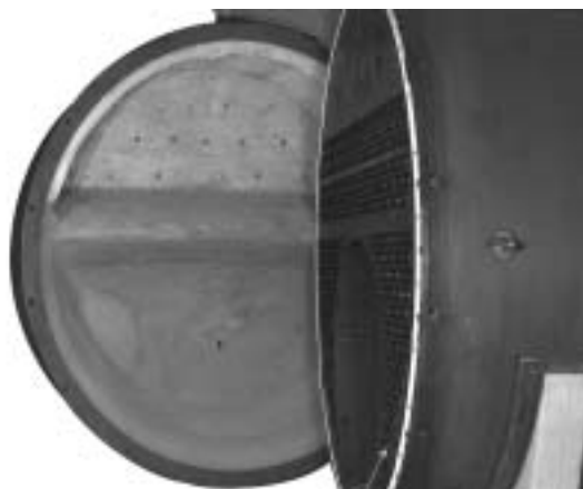
Figure 8-24: Rear Door Open
