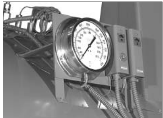
Figure: 6-5 Hot Water Controls
