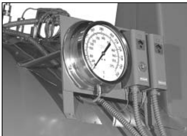
Figure: 1-11 Water Temperature Gauge
