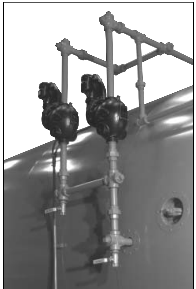
Figure: 1-8 Auxiliary Low Water Cut Off
