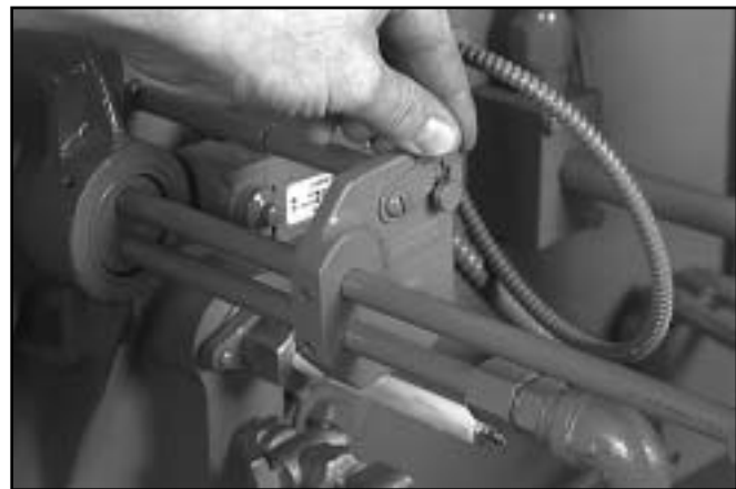
Figure: 6-18 Oil Gun Locked Out
