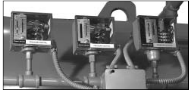
Figure: 6-7 Steam Operating Controls
